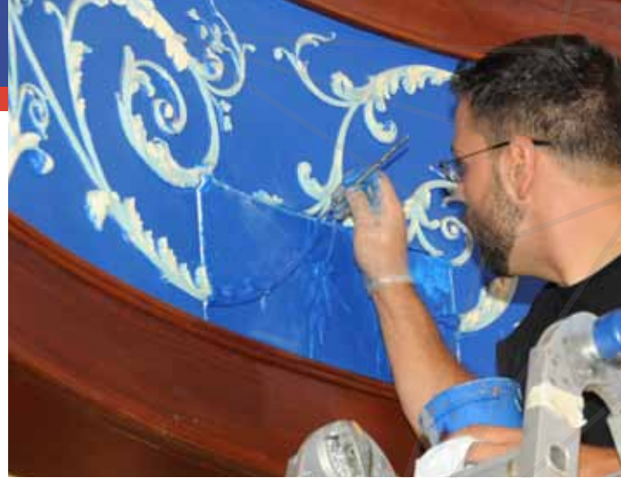
A SKILLED ARTISAN CAREFULLY REPAIRS DECORATIVE PLASTER
