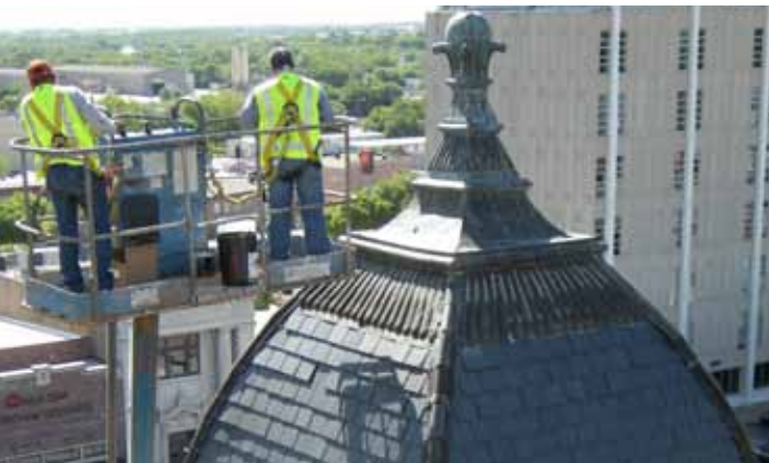
SLATE SHINGLES ARE REPLACED ON THE DOME
