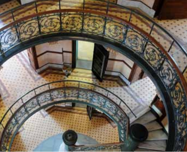
FULLY-RESTORED ORNATE RAILINGS IN THE CENTRAL STAIRCASE
