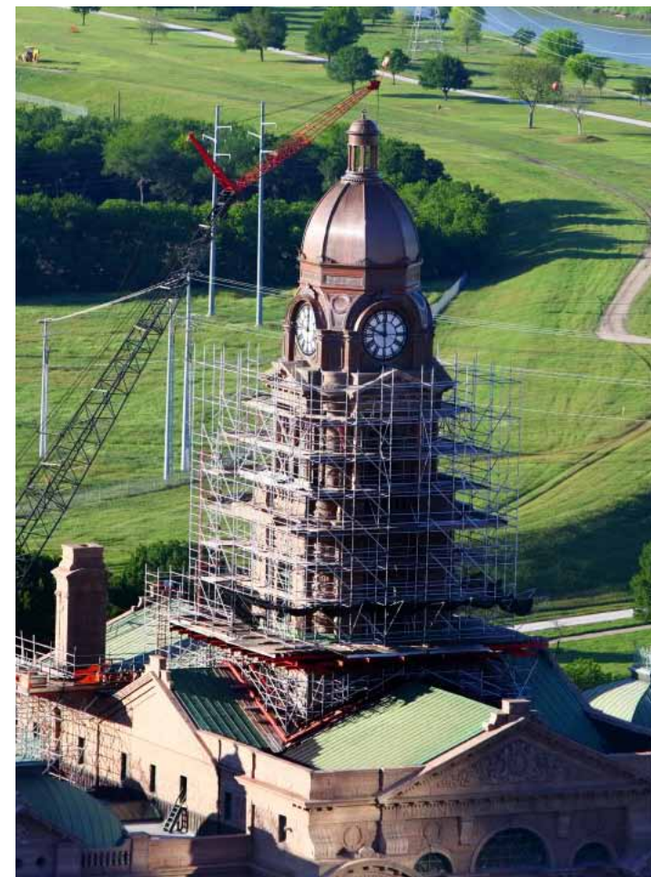
TARRANT COUNTY COURTHOUSE COPPER DOME WAS COMPLETELY REBUILT DURING RECENT RESTORATION EFFORTS
