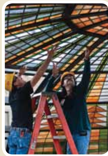
The glass dome will be restored in Houston's Harris County Courthouse.
