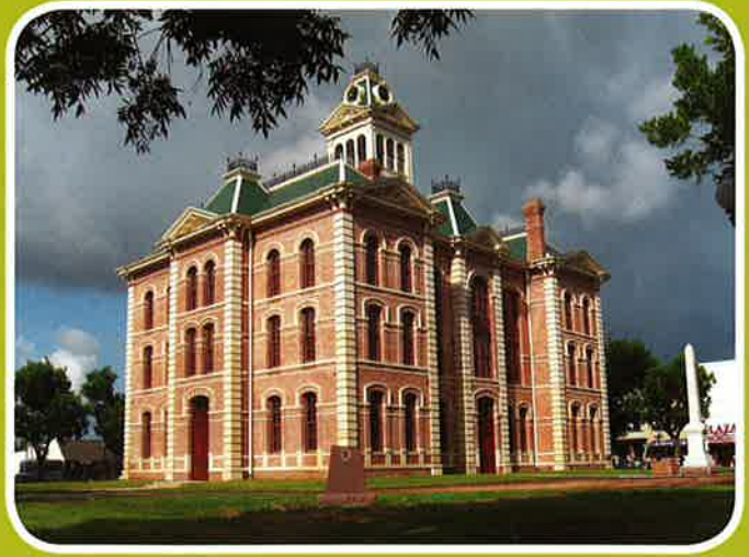
The project is considered one of the most dramatic restorations in the program.
