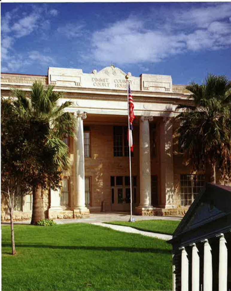
1926 Dimmit County Courthouse
