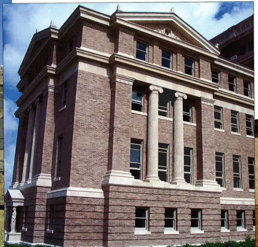
1914 Nueces County Courthouse
