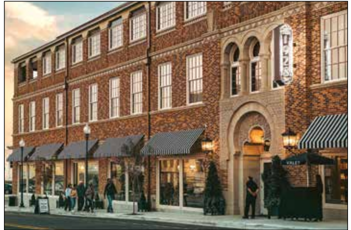
The Karem Shrine Temple in downtown Waco was rehabilitated as Hotel 1928 by the Magnolia team, utilizing state and federal historic preservation tax credits. Photo credit: Ryan LLC.
