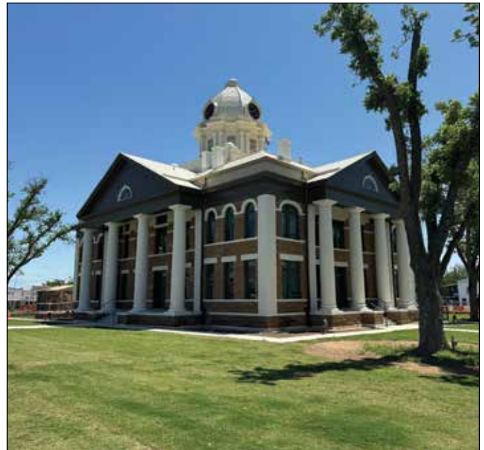
Following a 2021 arson fire, the Texas Legislature appropriated $6 million, the THC contributed a $4.1 million grant through the Texas Historic Courthouse Preservation Program, and other state and local organizations raised funds for a reconstruction of the Mason County Courthouse in Mason. It is slated to be rededicated on July 13, 2024. Photo courtesy of Architexas.
