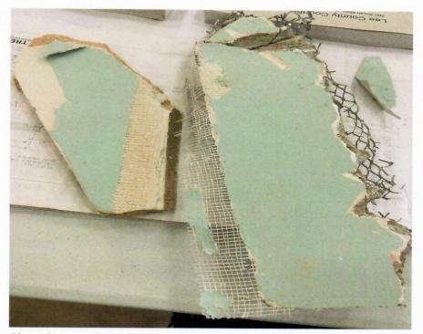
Photo shows condition and use of drywall tape at plaster interfaces. The photo on the right illustrates the use of drywall muds on gypsum plaster and typical thickness of applications.
