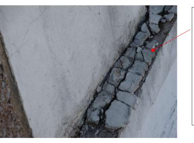
Mortar joint to be repointed and missing weather cap.
