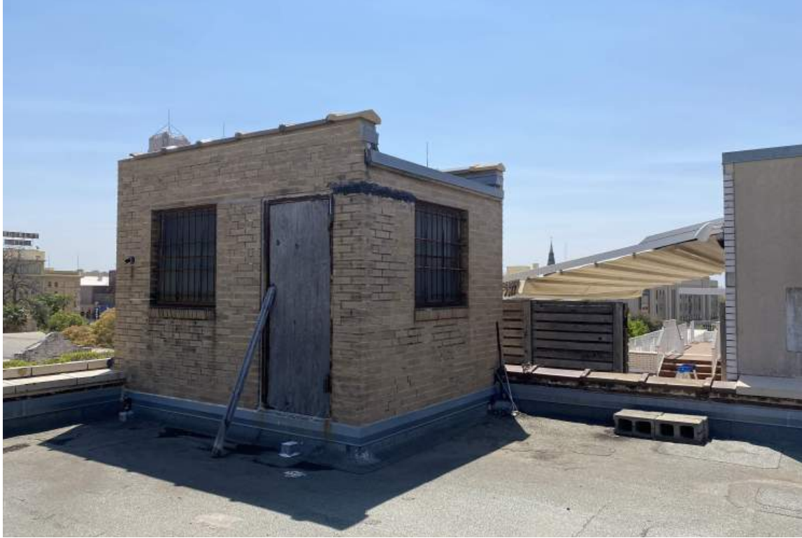
18. Existing Conditions: Woolworth Building utility house, view looking southeast.
