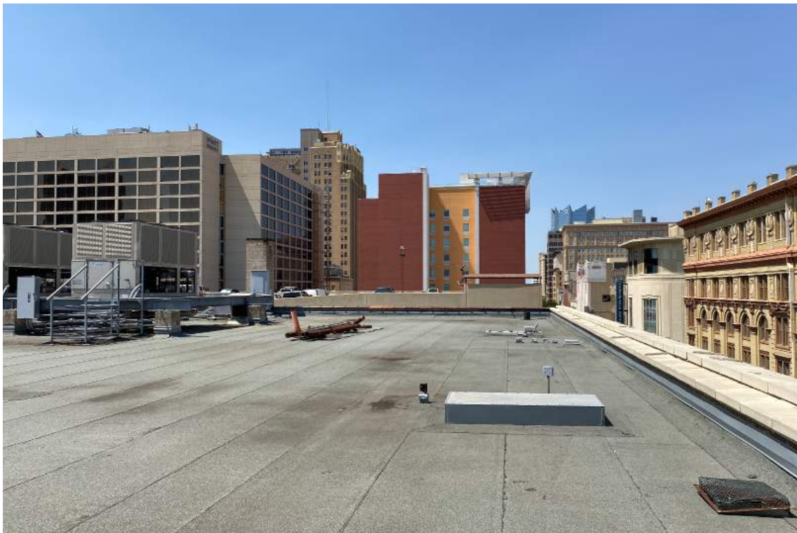
17. Existing Conditions: Woolworth Building Roof, view from northeast corner looking west.
