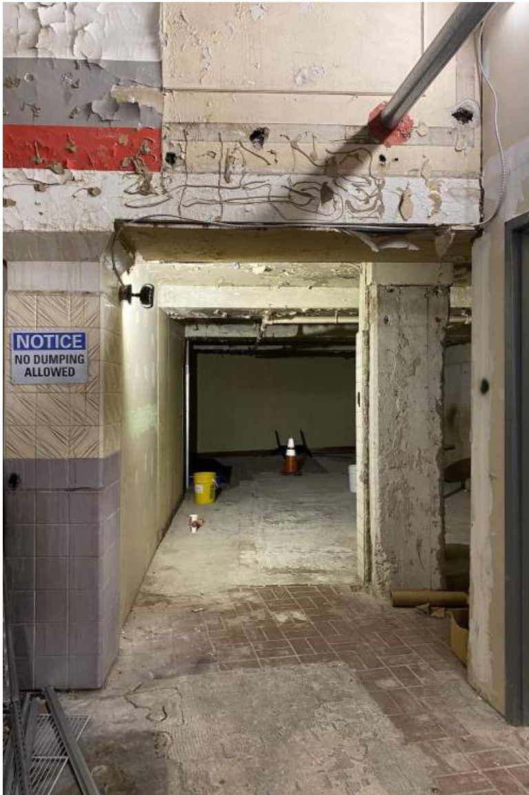
41. Existing Conditions: Woolworth Building Interior first floor, view looking south.
