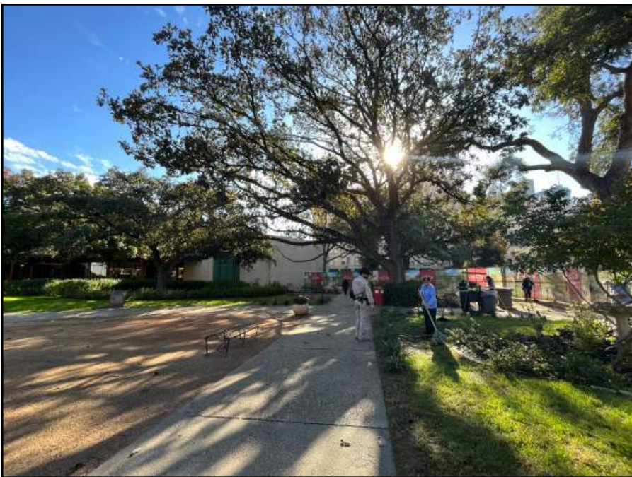
I- View looking southeast towards Bonham St. Construction fencing has been erected for future Texas Cavaliers Education Center.
