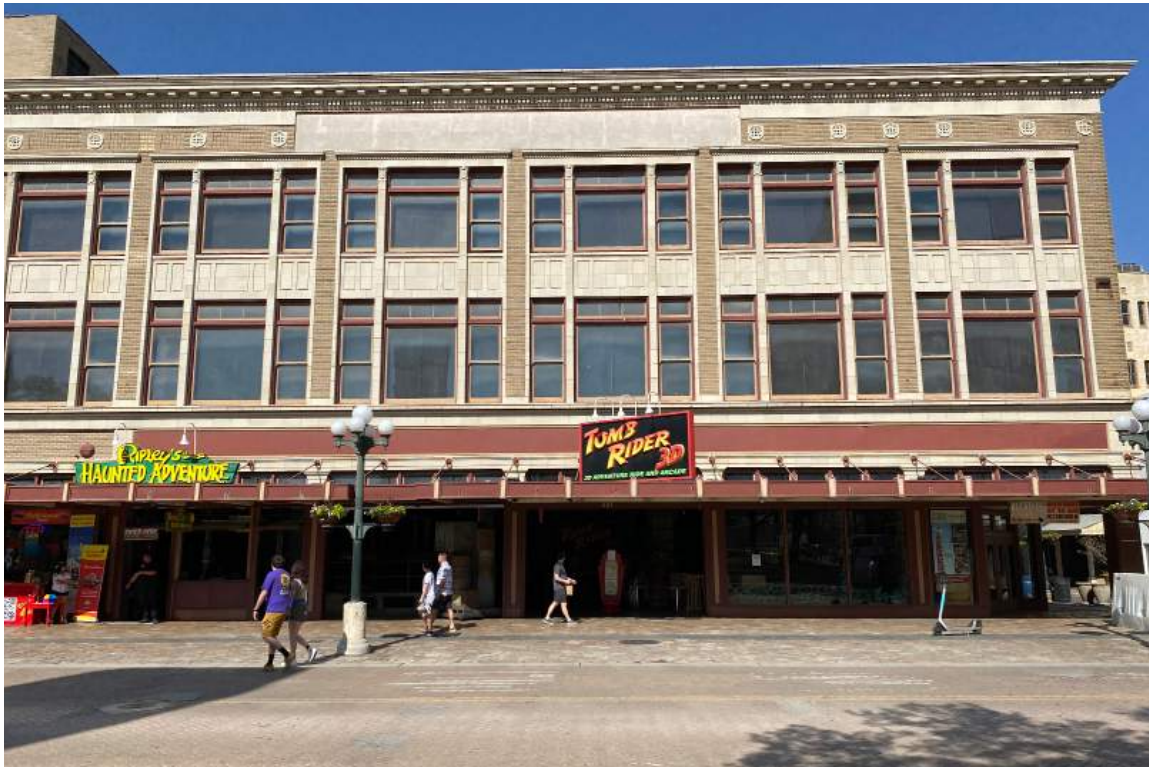
02. Existing Conditions: Woolworth Building Exterior, from Alamo Plaza looking west.
