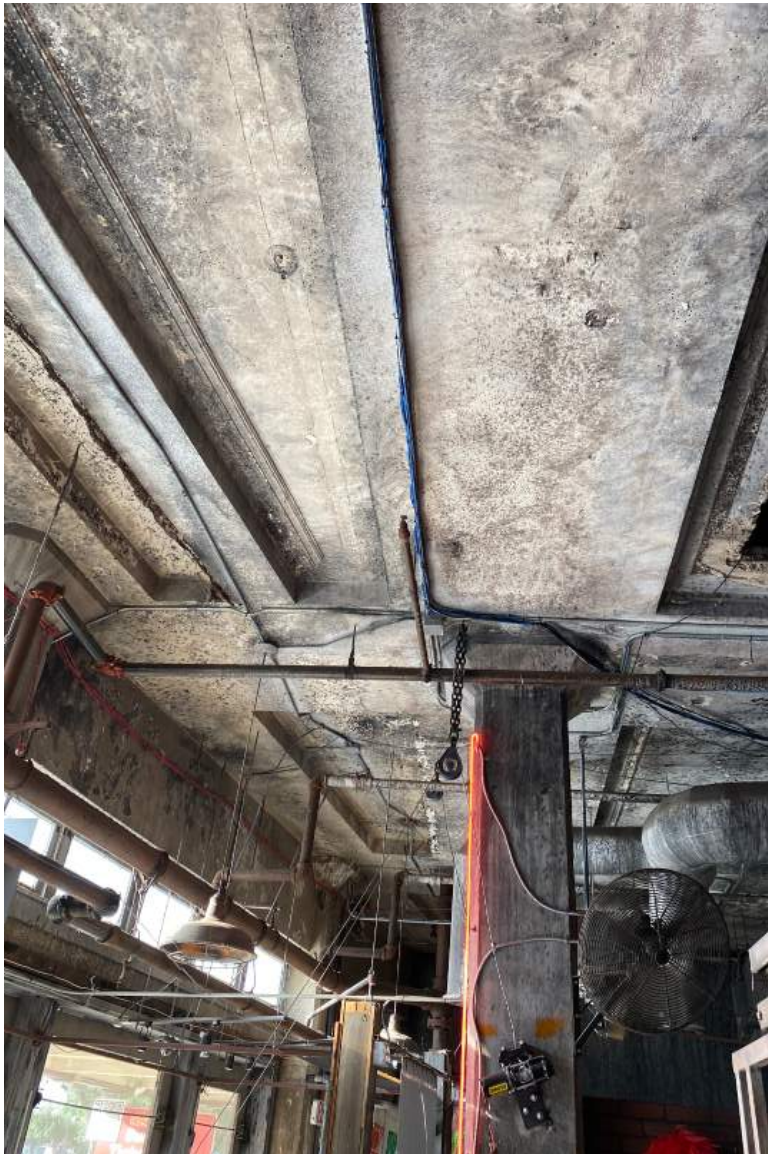
32. Existing Conditions: Woolworth Building Interior first floor, view up looking south.
