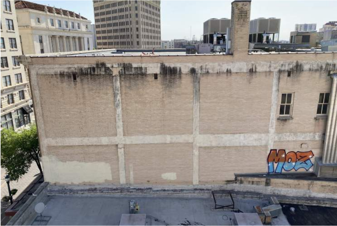
12. Existing Conditions: Woolworth Building Exterior, from west alley looking east.
