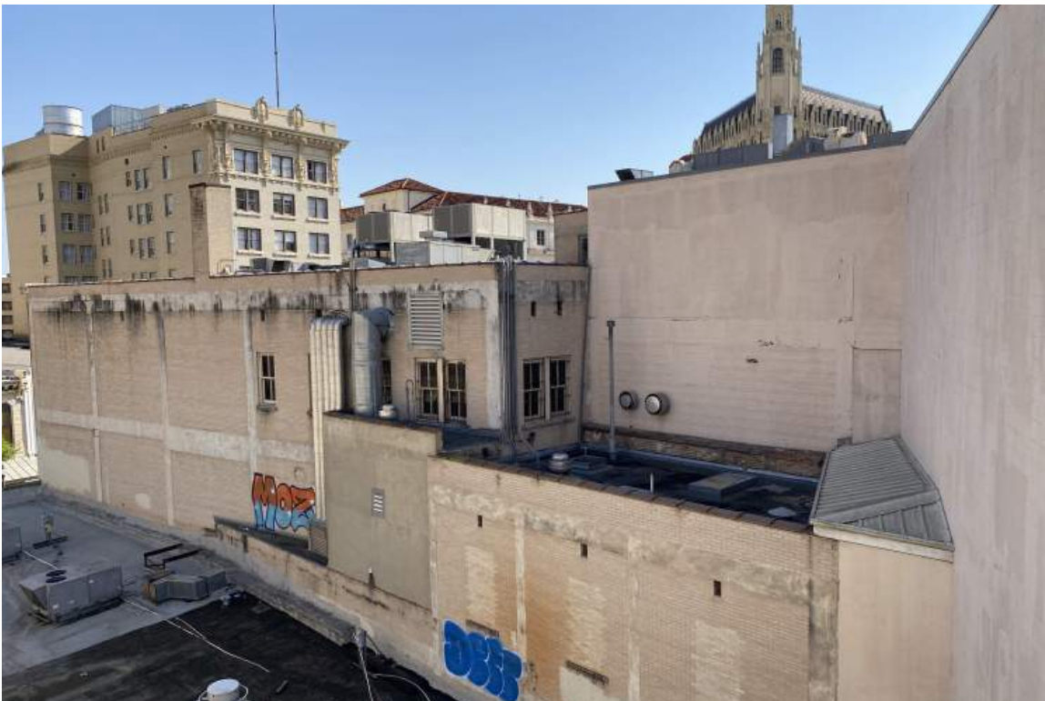
13. Existing Conditions: Woolworth Building Exterior, from west alley looking northeast.
