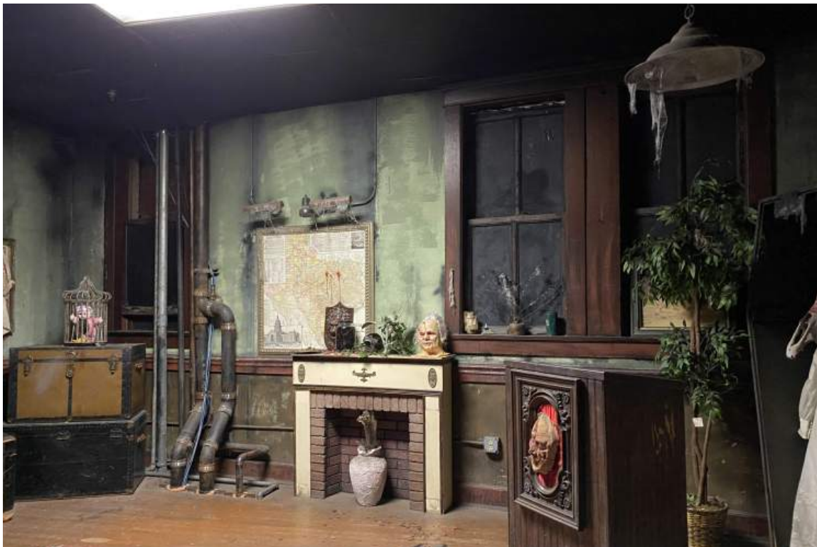
53. Existing Conditions: Woolworth Building Interior third floor, view looking south.
