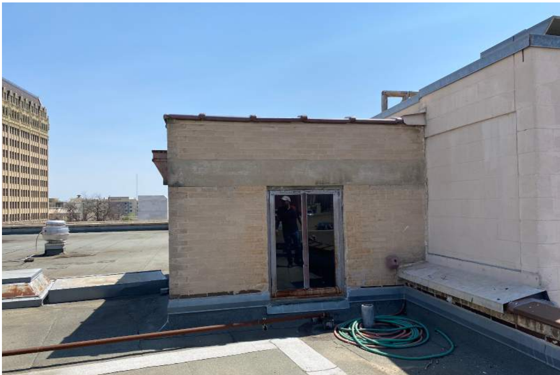
19. Existing Conditions: Woolworth Building elevator penthouse, view looking east.
