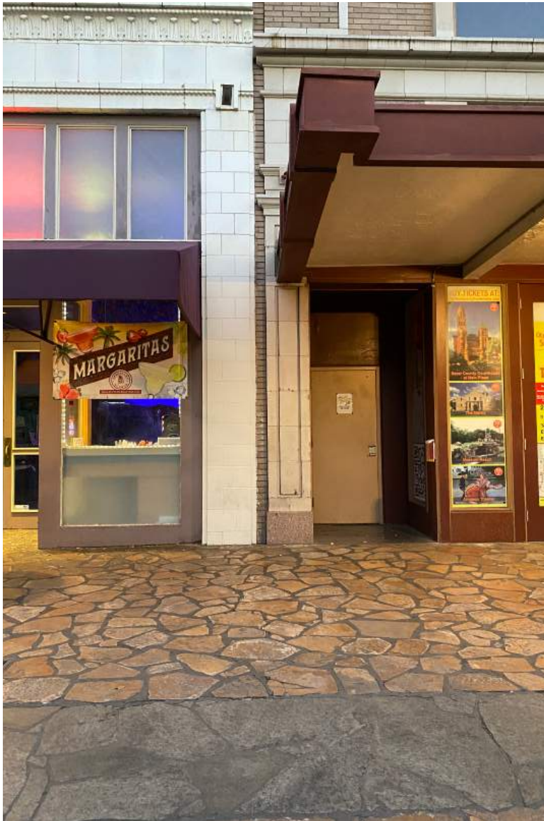
03. Existing Conditions: Woolworth Building Exterior, from Alamo Plaza looking west.
