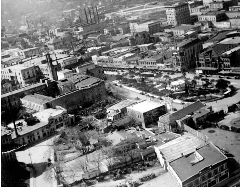
Aerial View looking Southwest - 1919 UTSA Digital Archive
