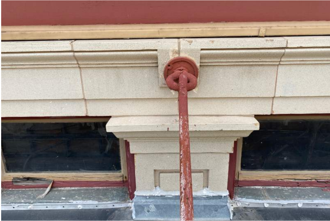
05. Existing Conditions: Woolworth Building Canopy detail, Houston Street side looking south.
