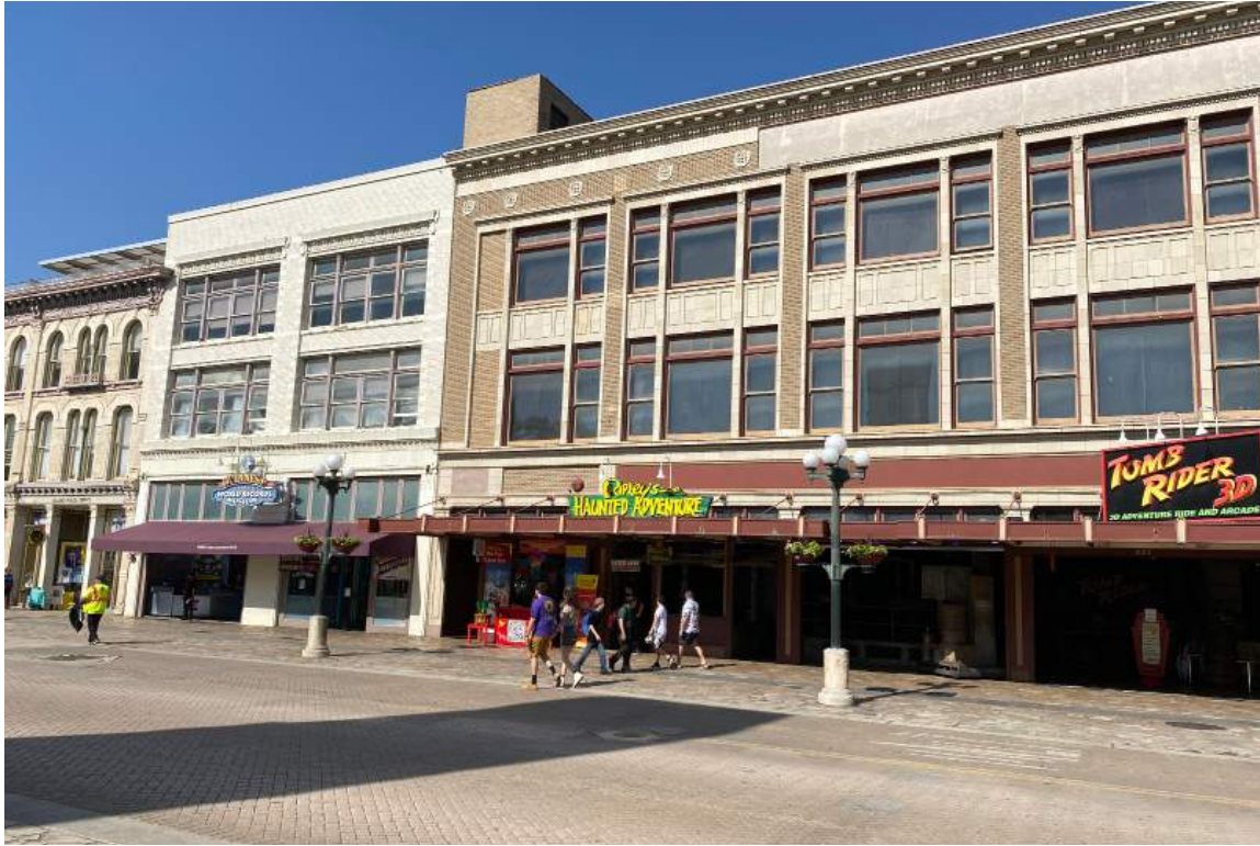
01. Existing Conditions: Woolworth Building Exterior, from Alamo Plaza looking west.
