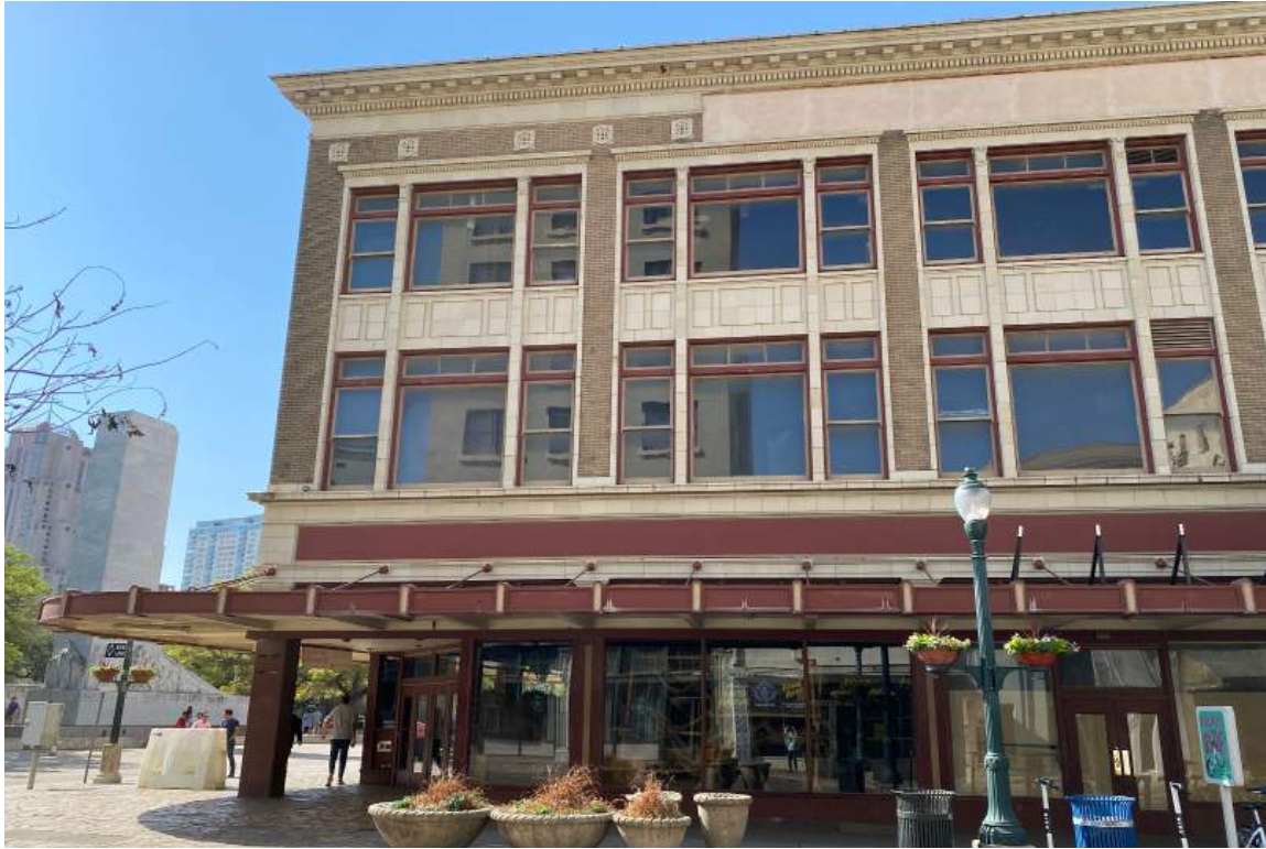
07. Existing Conditions: Woolworth Building Exterior, from Houston Street looking south.
