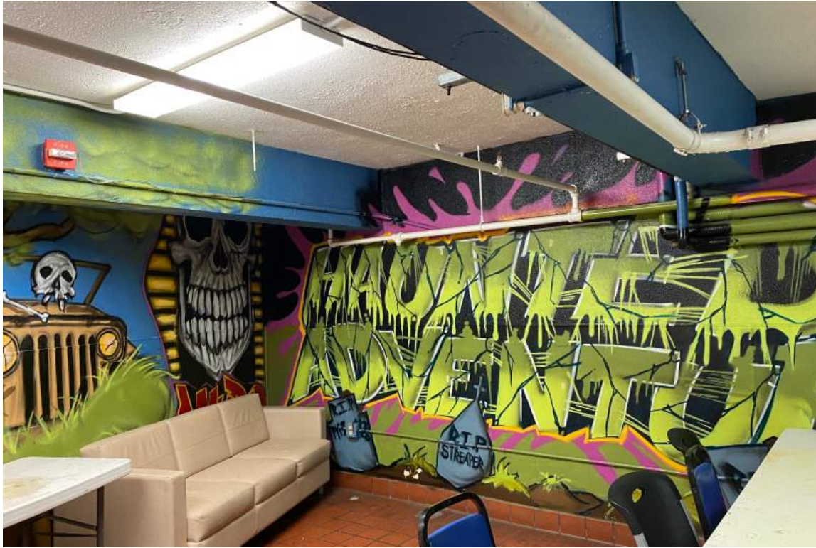
43. Existing Conditions: Woolworth Building Interior mezzanine, view looking south.
