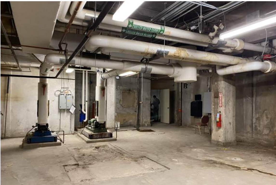
22. Existing Conditions: Woolworth Building Interior basement, view looking south.
