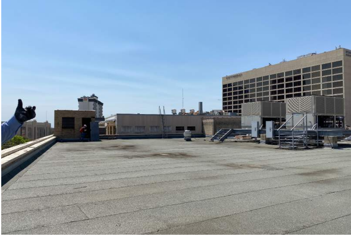
16. Existing Conditions: Woolworth Building Roof, view from northeast corner looking south.
