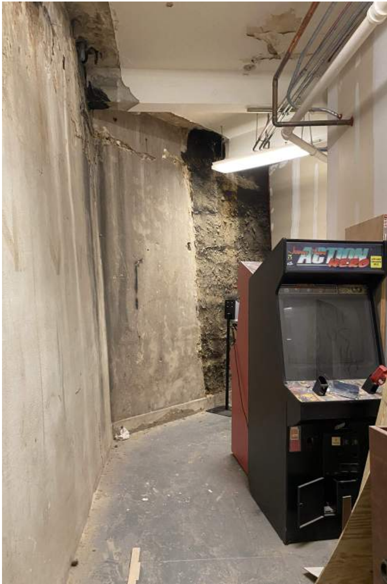
26. Existing Conditions: Woolworth Building Interior basement, view looking east.
