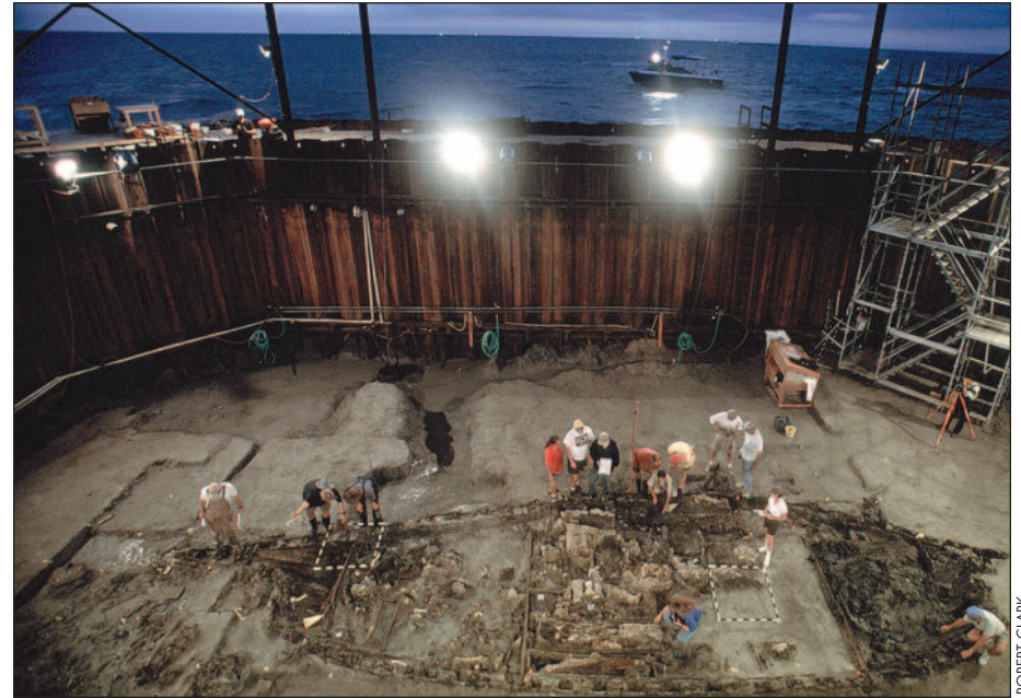
In 1996, a giant cofferdam was built around the Belle and the water inside pumped out, allowing an almost dry-land excavation. This photo shows the shipwreck as it was just beginning to be uncovered from the muddy bottom of Matagorda Bay.
