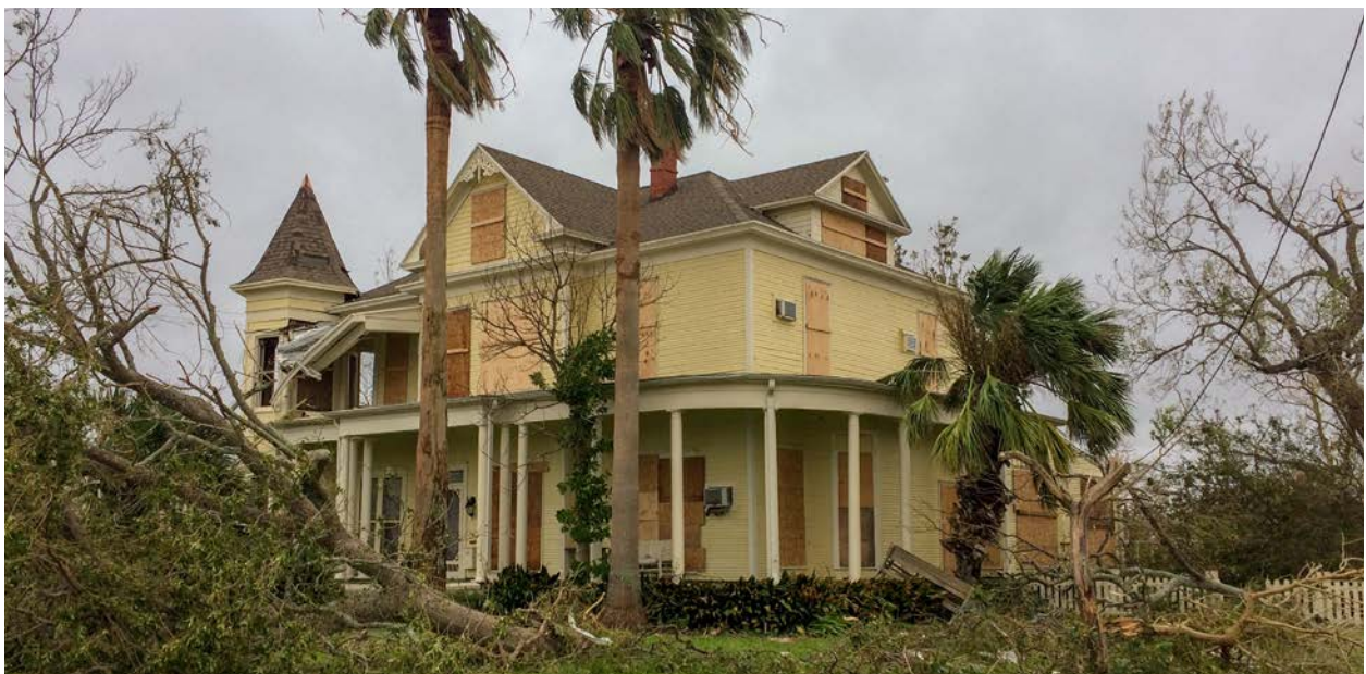
LEOPOLD M. BRACHT HOUSE, POST HURRICANE HARVEY, ROCKPORT, TEXAS
