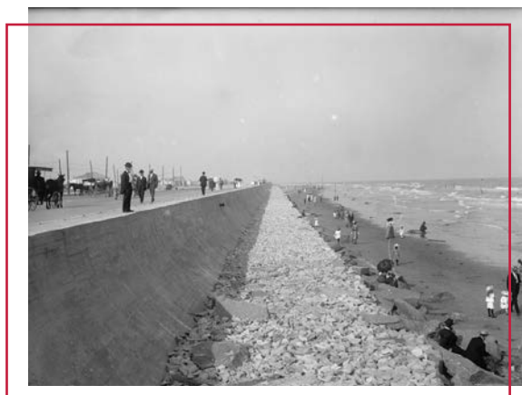
GALVESTON SEAWALL, CIRCA 1920, LIBRARY OF CONGRESS
