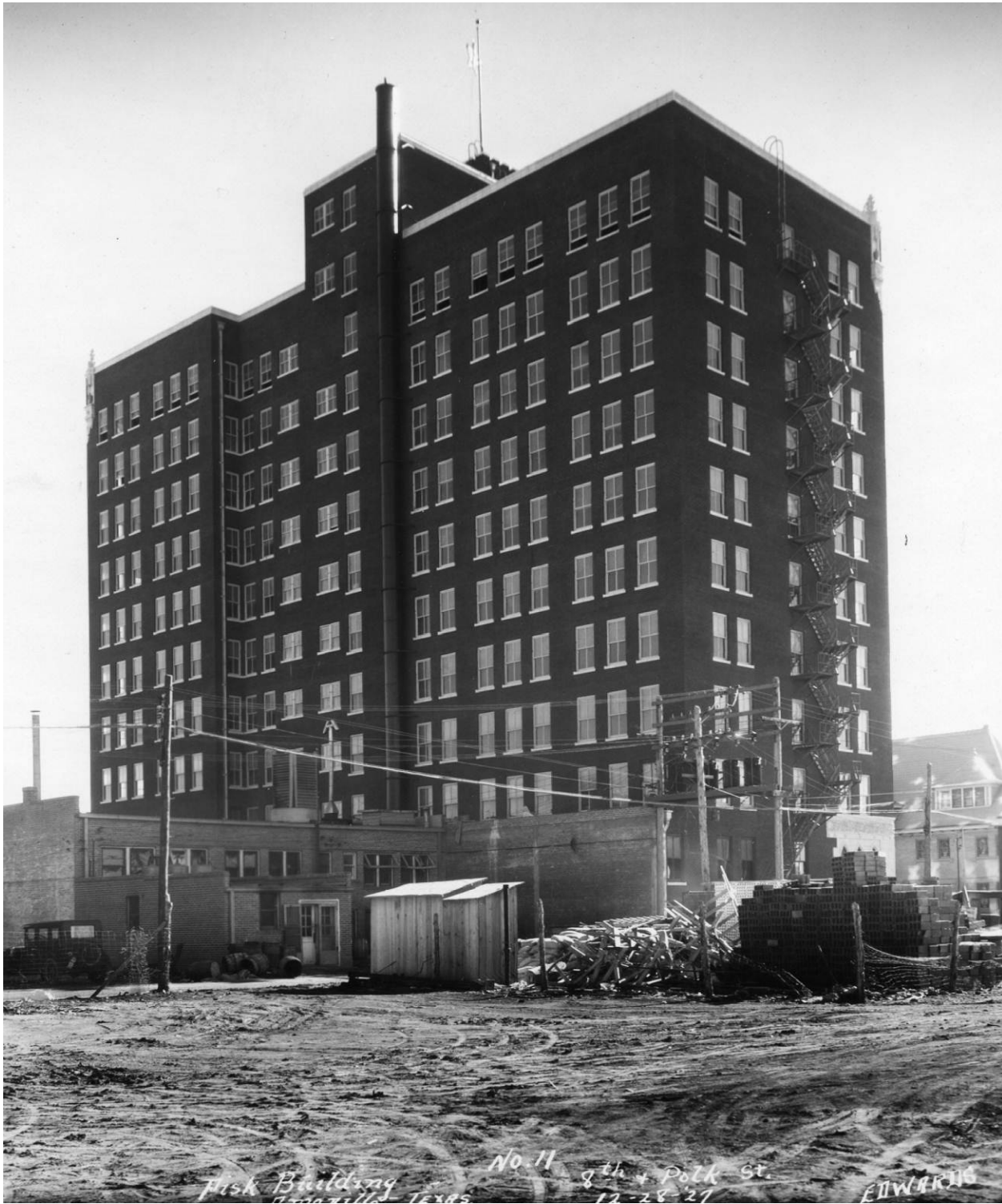
Façade at Northwest Corner, 1928.
