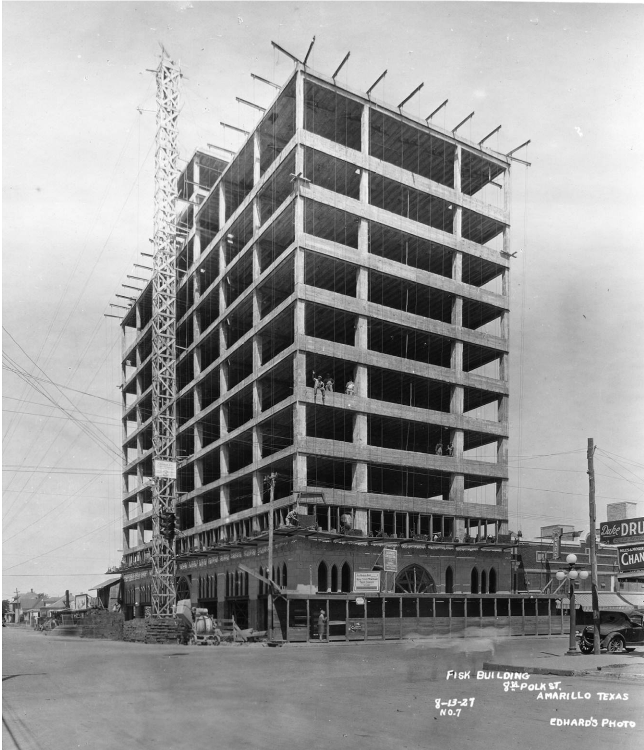
Stone Veneer Construction, 1927.
