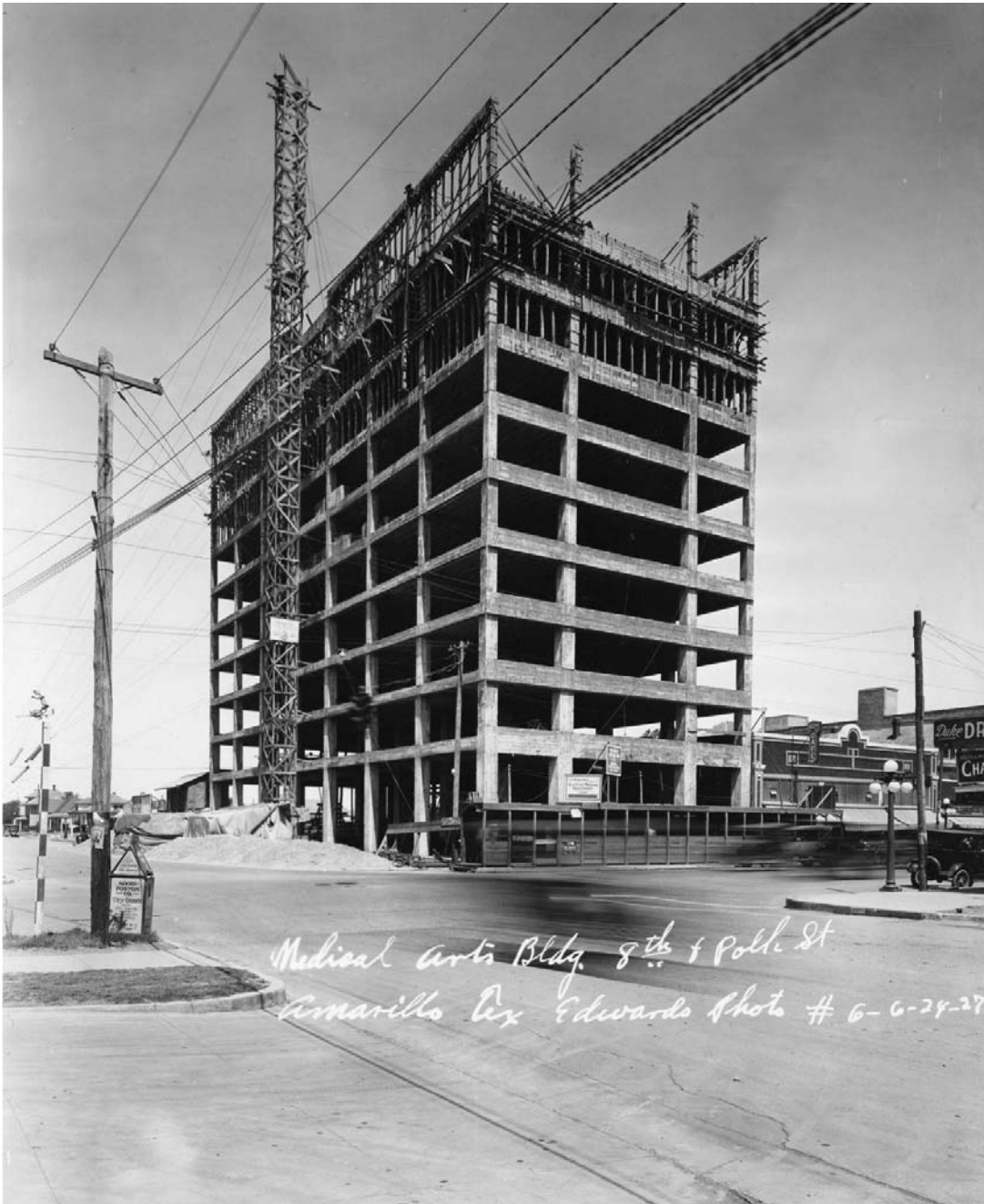
Structural Concrete Framing, 1927.
