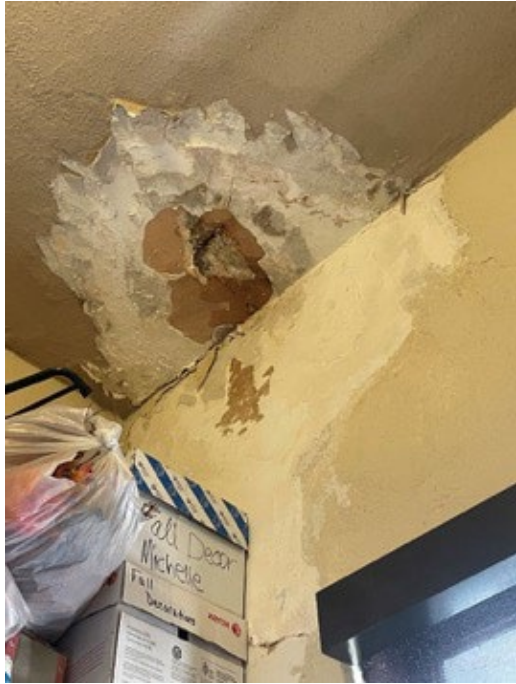
Fourth Floor East Elevation - Exhibit Room
