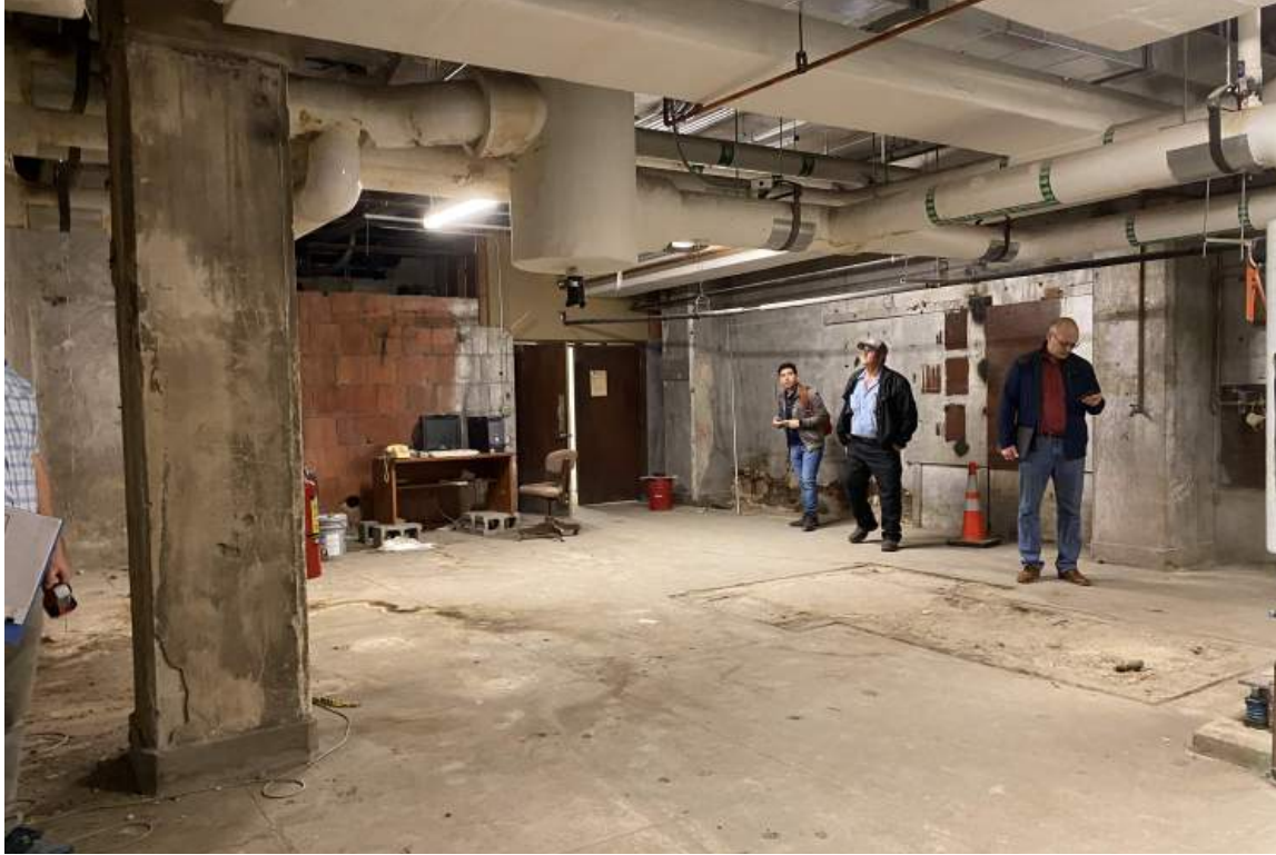
21. Existing Conditions: Woolworth Building Interior basement, view looking north.
