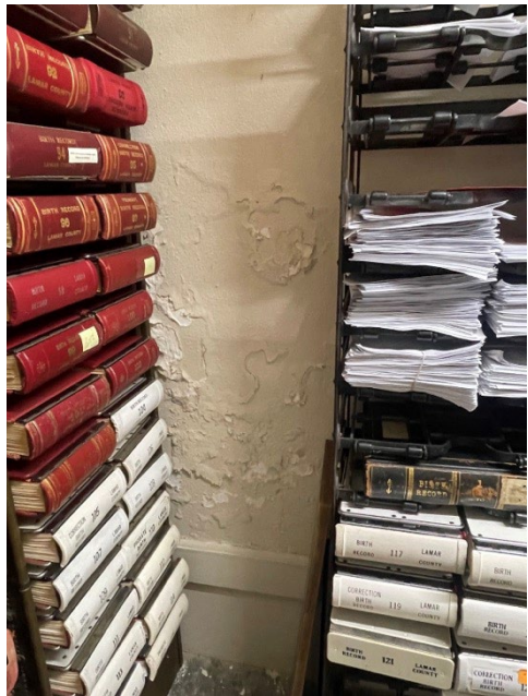
Annex North Elevation - County Clerk Dark Room
