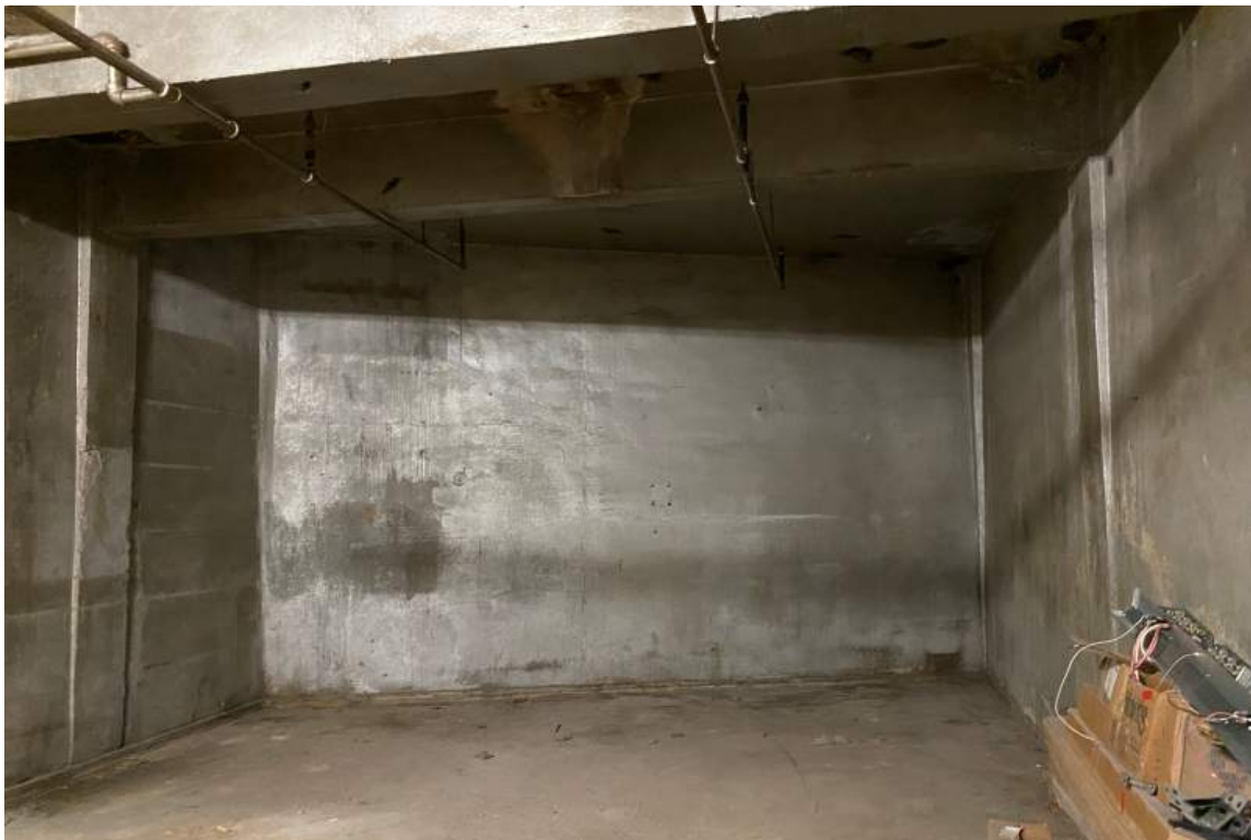
24. Existing Conditions: Woolworth Building Interior basement, view looking south.
