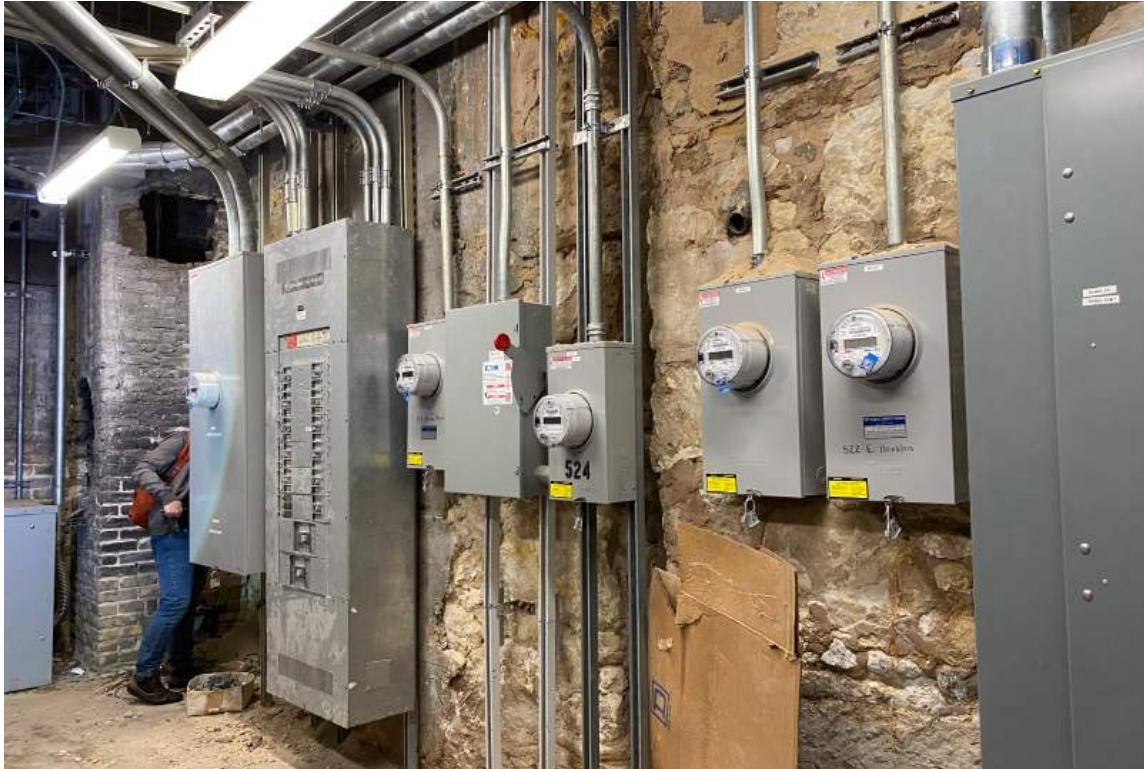
23. Existing Conditions: Woolworth Building Interior basement, view looking southwest.
