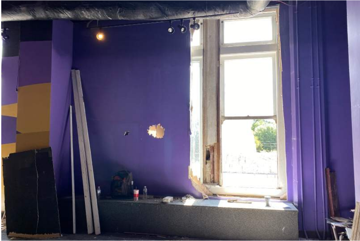
46. Existing Conditions: Woolworth Building Interior second floor, view looking east.
