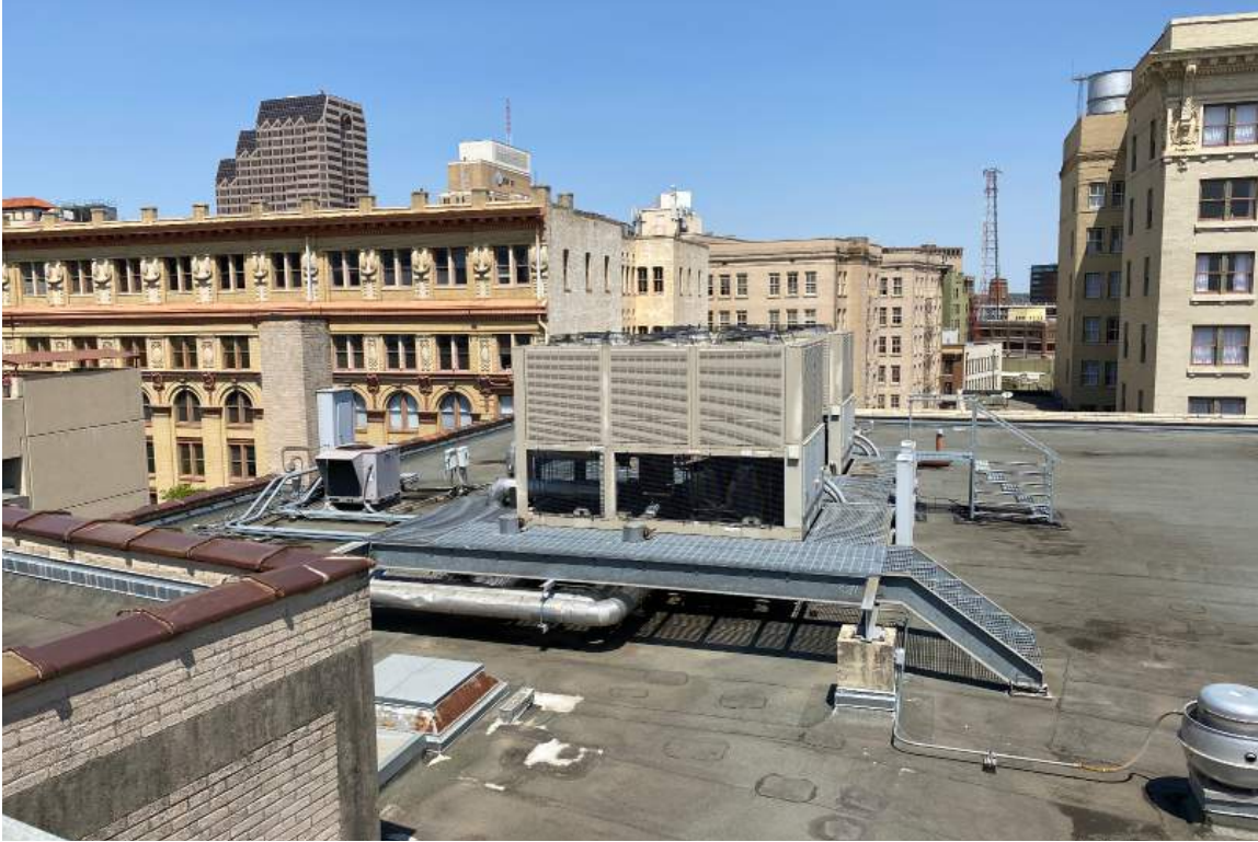
14. Existing Conditions: Woolworth Building Roof, view from south end looking northwest.
