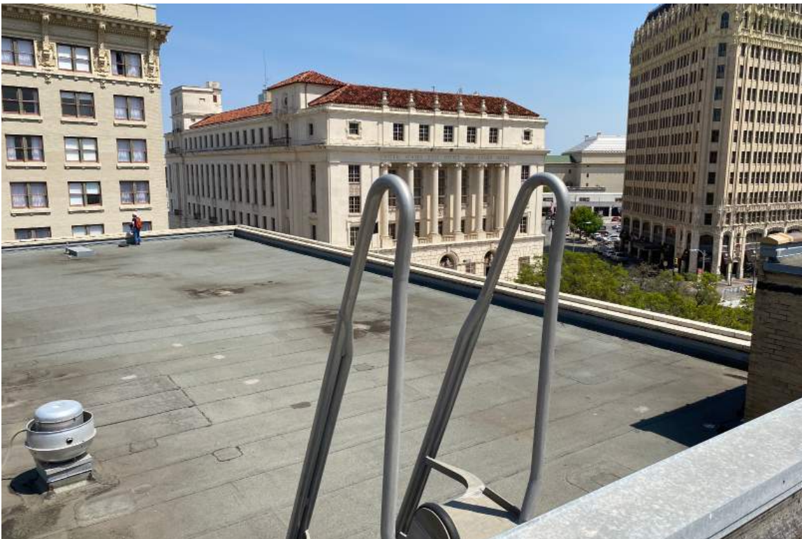
15. Existing Conditions: Woolworth Building Roof, view from south end looking northeast.
