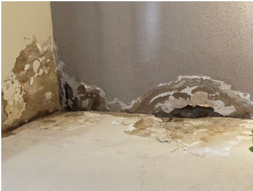
Fourth Floor East Elevation - Exhibit Room
