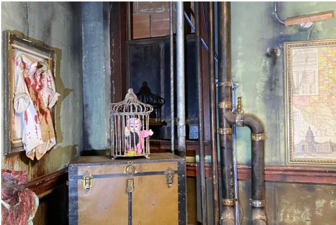
55. Existing Conditions: Woolworth Building Interior third floor, view looking south.
