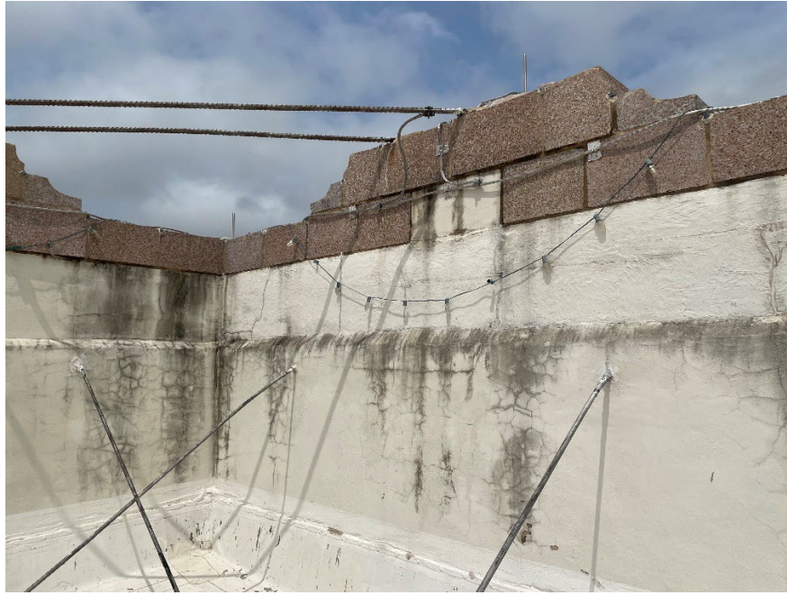
Lamar County Courthouse Roof - Northeast
