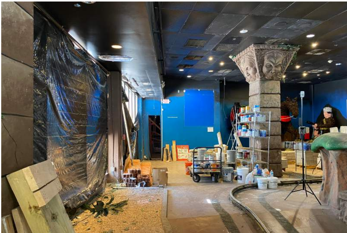
37. Existing Conditions: Woolworth Building Interior first floor, view looking south.
