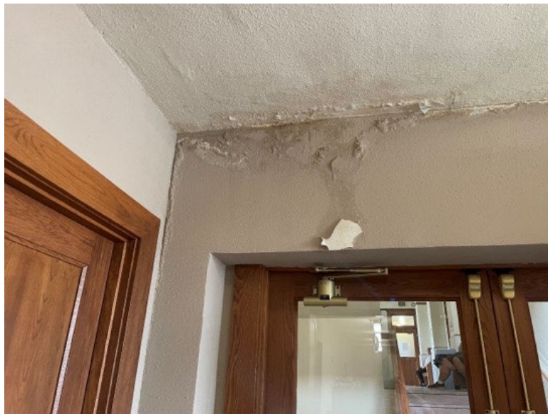
Annex East (Courthouse West) Elevation - Service Room
