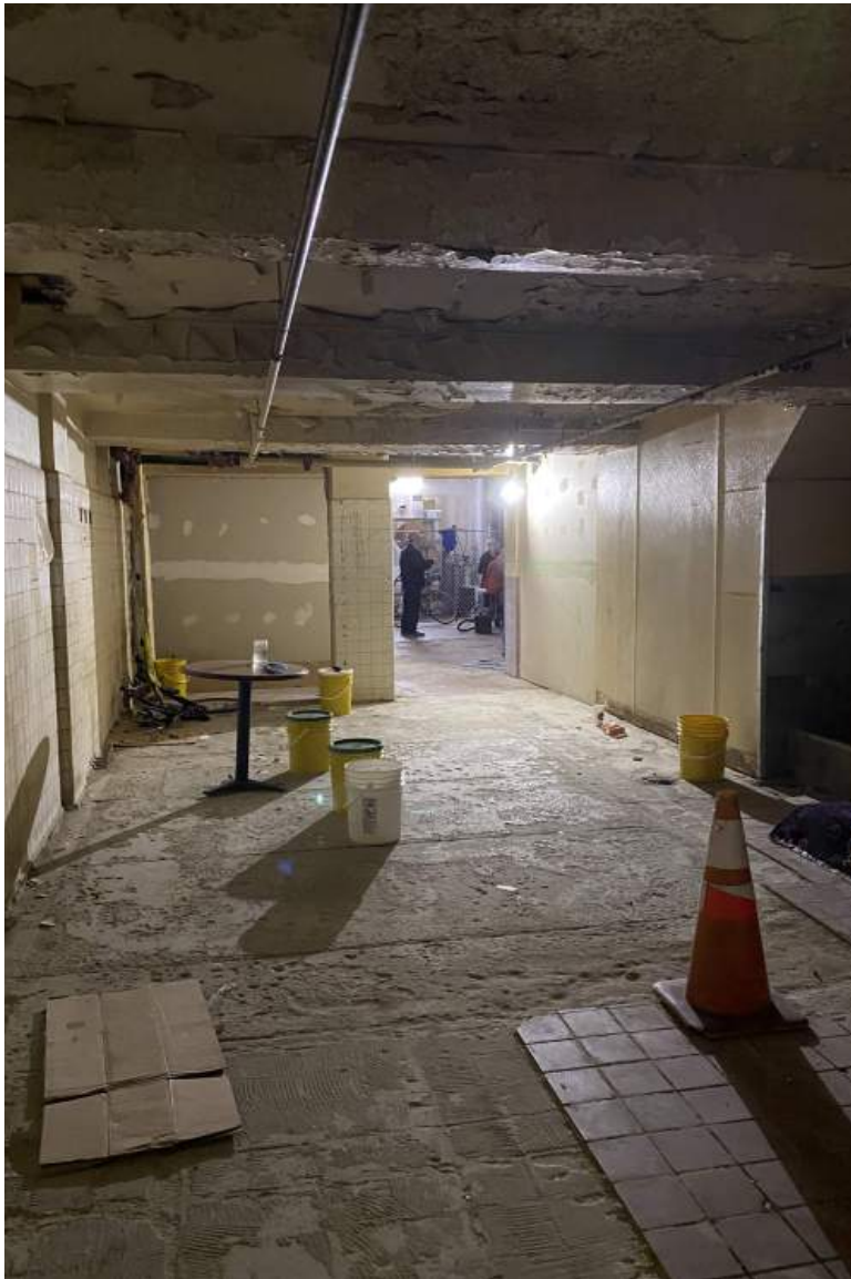
42. Existing Conditions: Woolworth Building Interior first floor, view looking north.
