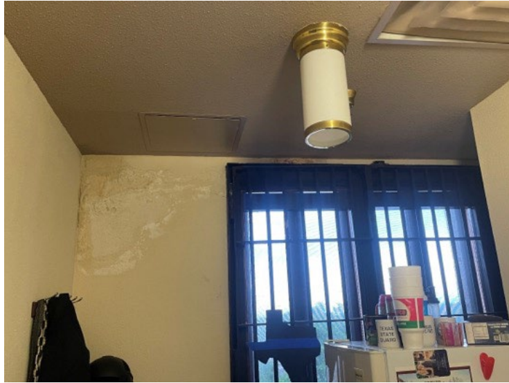
Fourth Floor West Elevation – County Court Workroom
