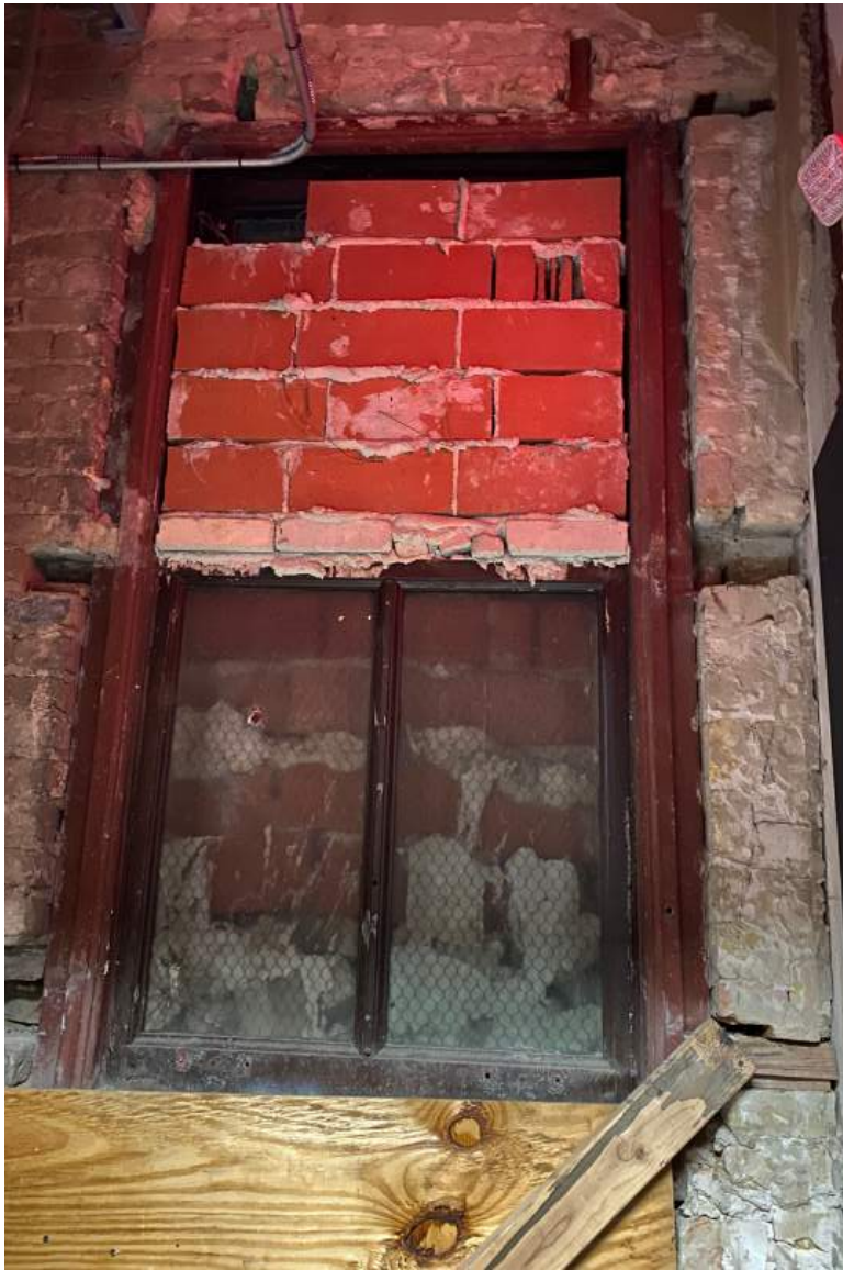
51. Existing Conditions: Woolworth Building Interior second floor, view of metal window.
