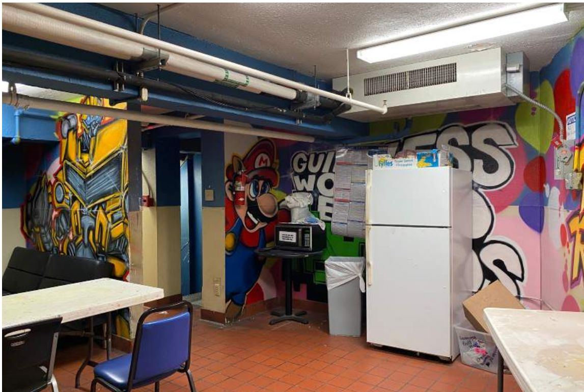
44. Existing Conditions: Woolworth Building Interior mezzanine, view looking north.
