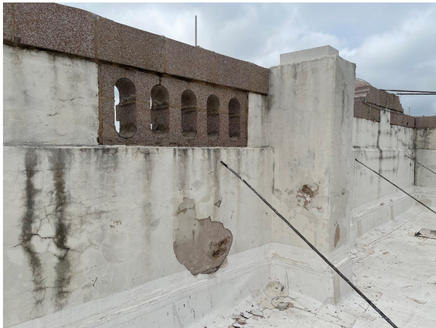
Lamar County Courthouse Roof - West
