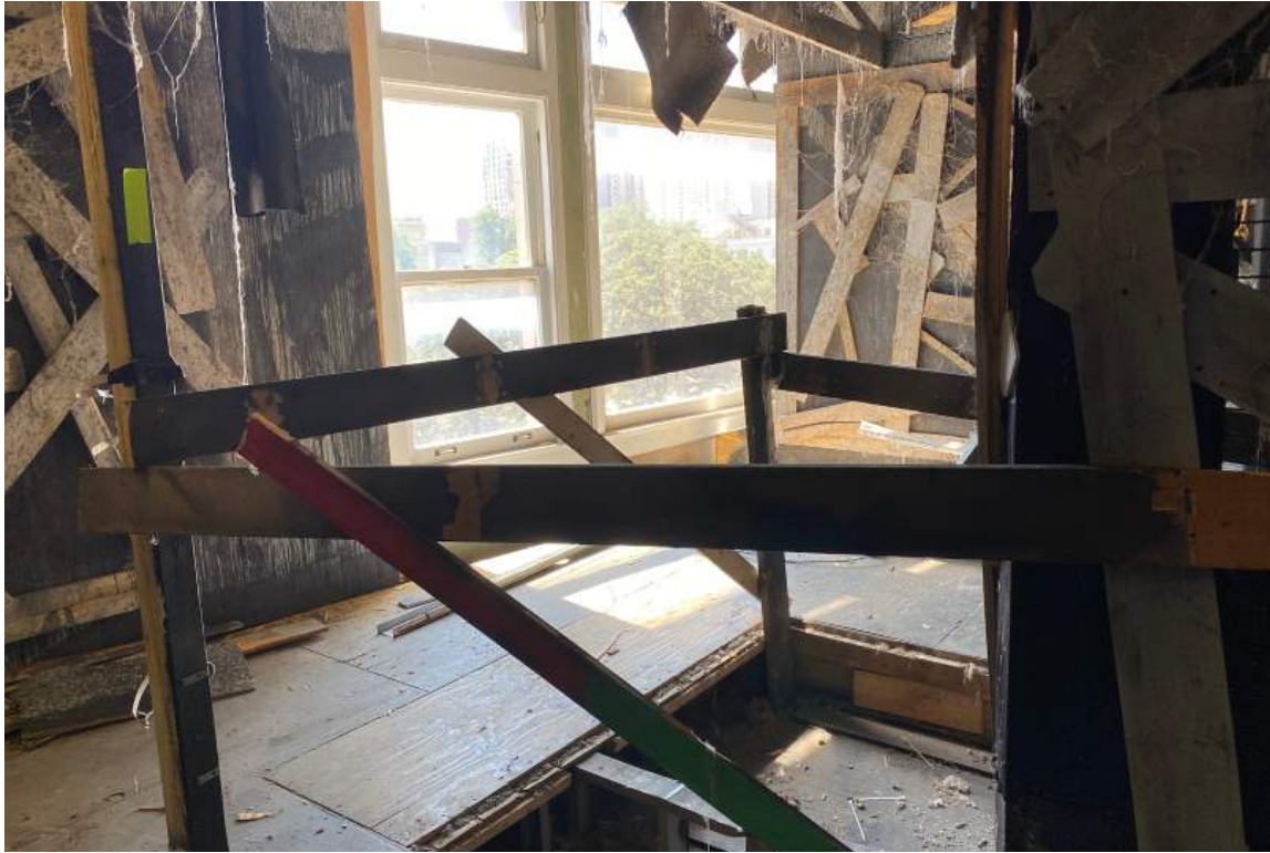
54. Existing Conditions: Woolworth Building Interior third floor, view northeast.
