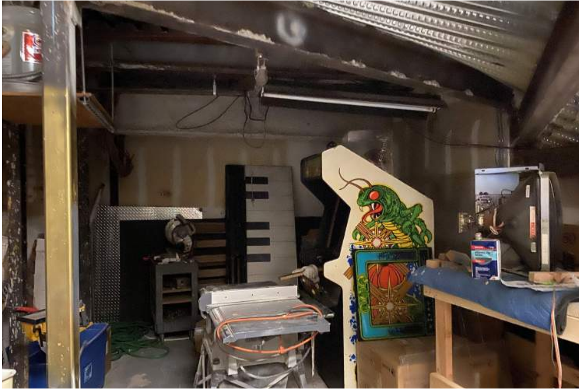
27. Existing Conditions: Woolworth Building Interior basement, view looking south.
