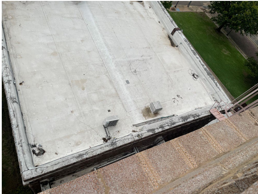
Lamar County Courthouse Annex Roof
