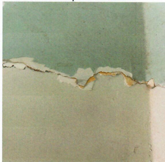
Photo shows thickness of the application
