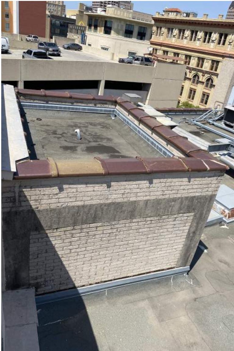
20. Existing Conditions: Woolworth Building elevator penthouse, view looking west.
