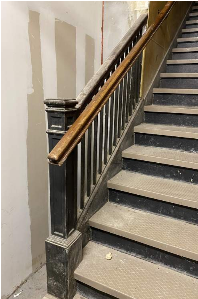
25. Existing Conditions: Woolworth Building Interior basement, view looking south.
