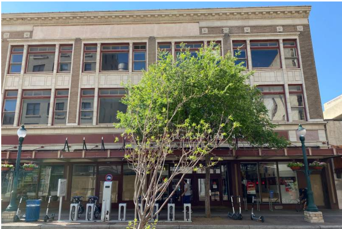
08. Existing Conditions: Woolworth Building Exterior, from Houston Street looking south.
