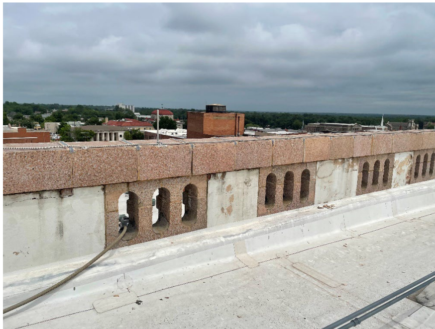
Lamar County Courthouse Roof - East
