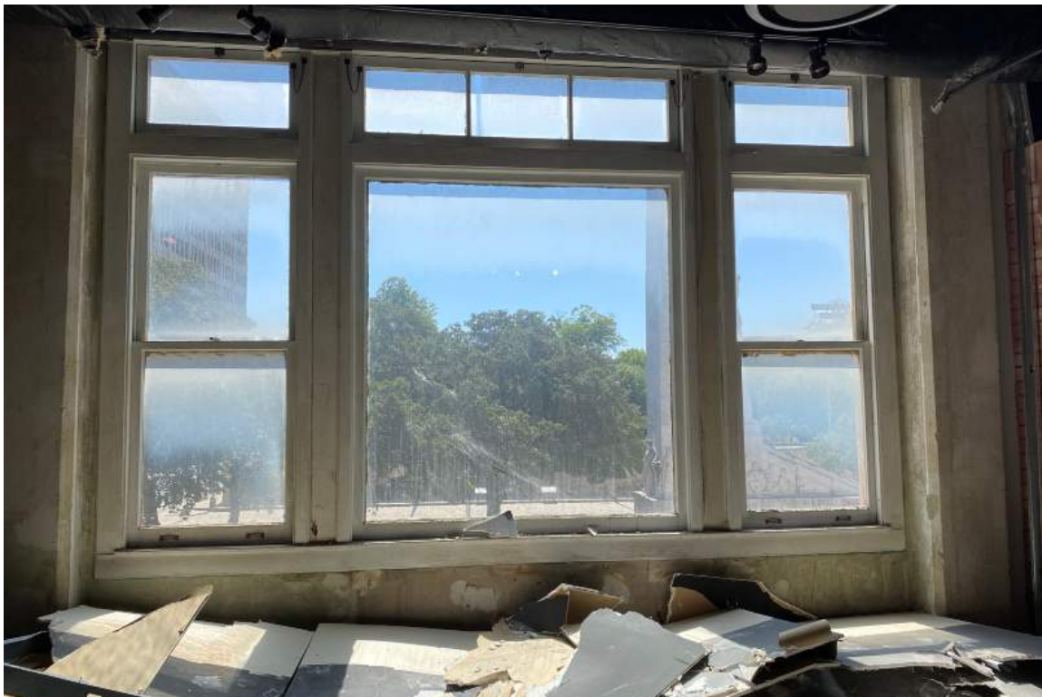
47. Existing Conditions: Woolworth Building Interior second floor, view looking north.
