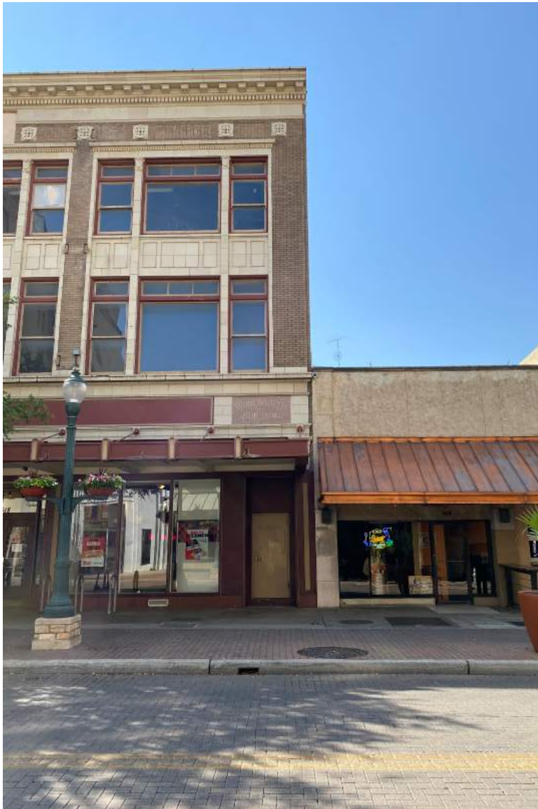
09. Existing Conditions: Woolworth Building Exterior, from Houston Street looking south.
