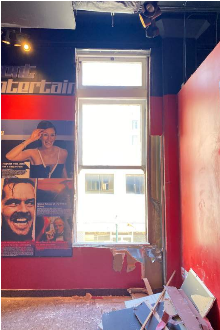
48. Existing Conditions: Woolworth Building Interior second floor, view looking north.
