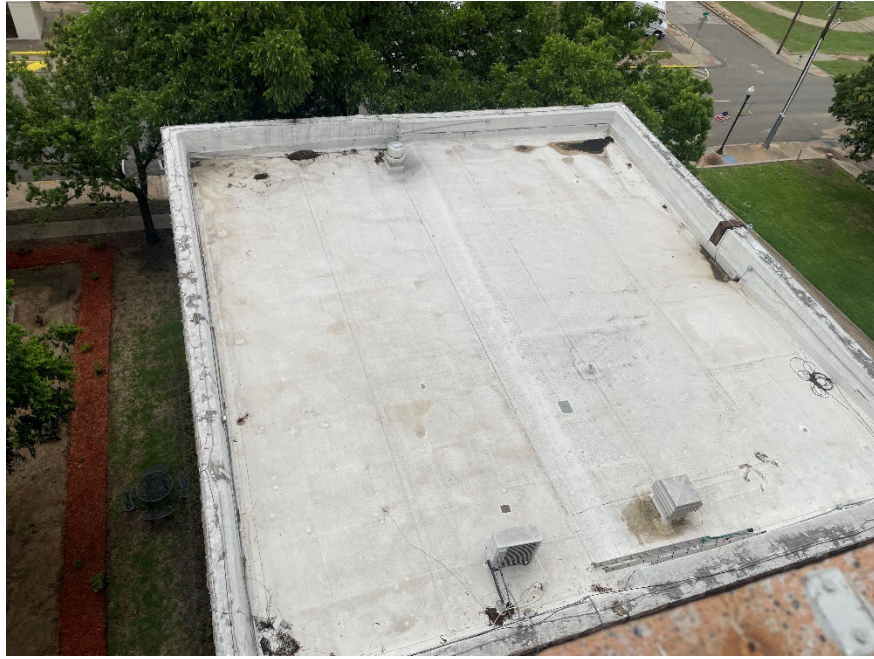
Lamar County Courthouse Annex Roof
