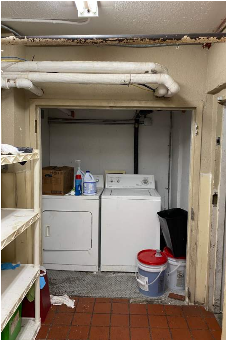
45. Existing Conditions: Woolworth Building Interior mezzanine, view looking north.
