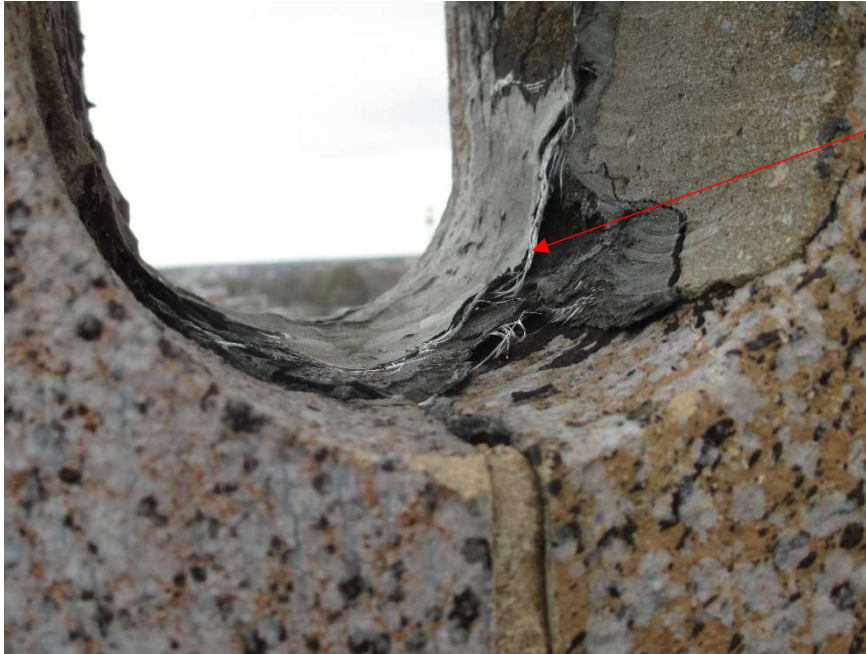
Concrete and asphalt removal from terra cotta openings
