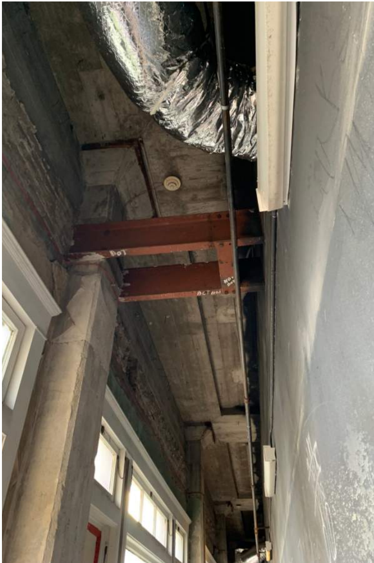
57. Existing Conditions: Woolworth Building Interior third floor, view up looking east.
