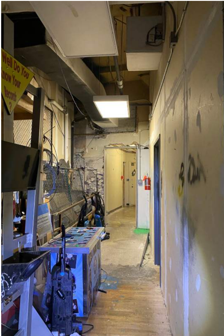
49. Existing Conditions: Woolworth Building Interior second floor, view looking south.
