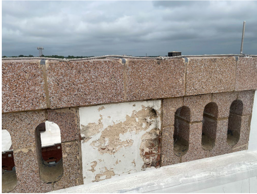
Lamar County Courthouse Roof - East
