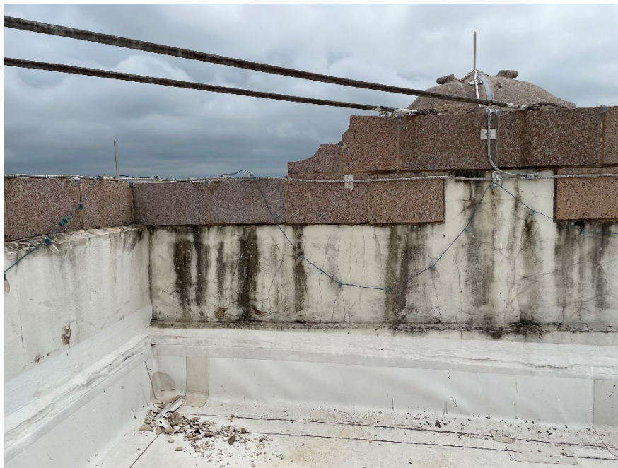
Lamar County Courthouse Roof - Southeast
