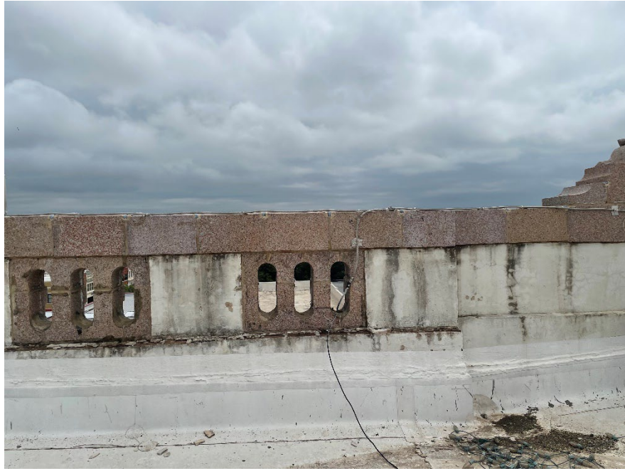
Lamar County Courthouse Roof - South
