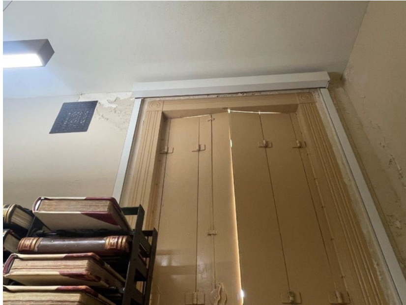
Annex North Elevation - County Clerk Dark Room
