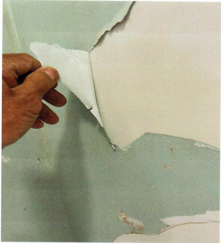
*Photo shows lack of paint bonding to drywall muds*
