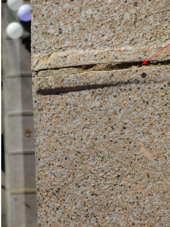
Mortar joint to be repointed and missing weather cap.
