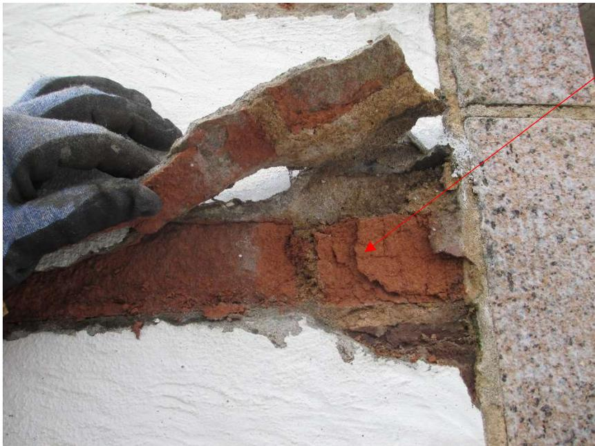
Damaged brick back-up covered by plaster/stucco.
