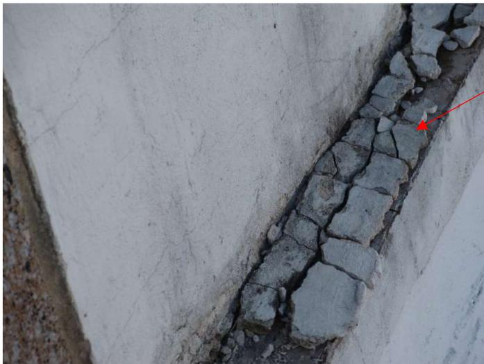
Deteriorated Plaster/stucco ledge needing repairs.
