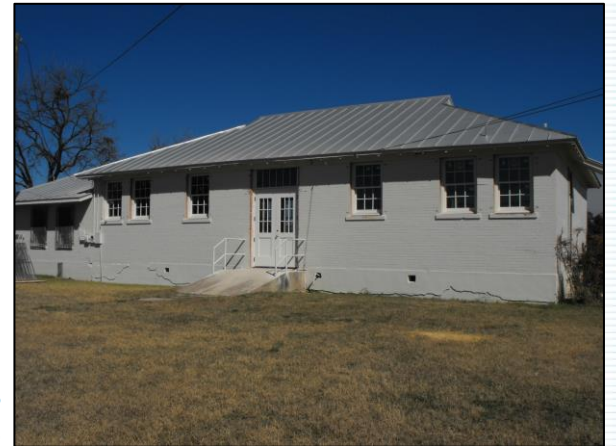
Architecture Development, FY 2015 - $15,000, Nicolas Street School, Uvalde
